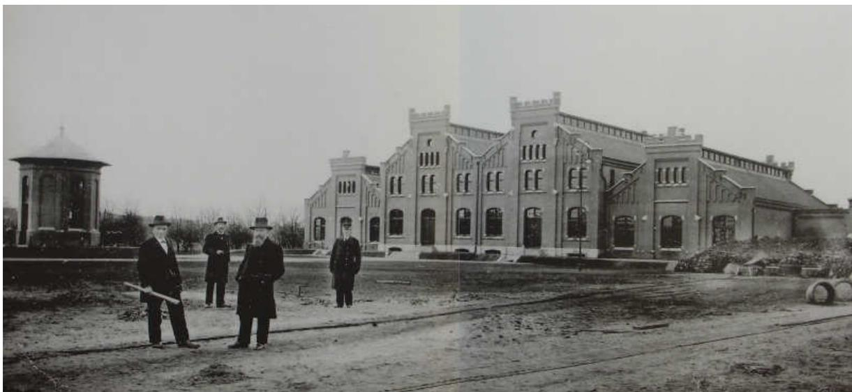
The Pump Engine Building was opened in 1900. Until 1941, it used (seven) steam engines; these were then replaced by electric motors.
